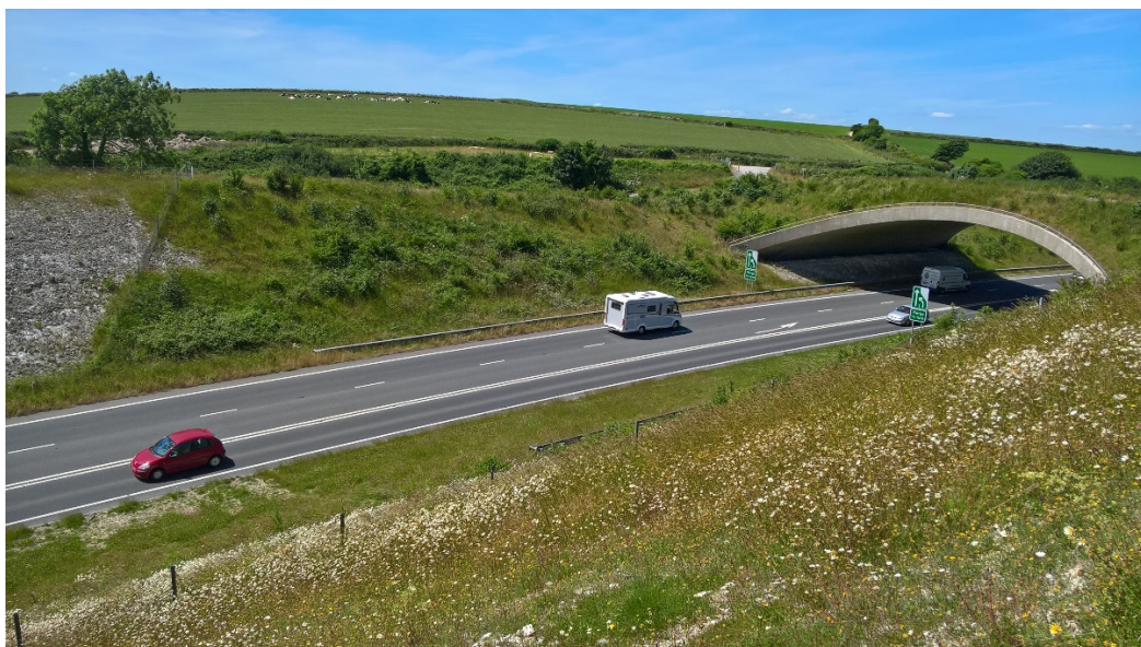
Example of overbridge spanning the dual carriageway, Weymouth relief road scheme
