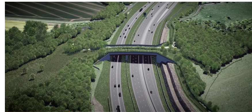
Figure 37. View south-west towards Gloucestershire Way crossing from south (above) and north (below) (Highways Agency).
