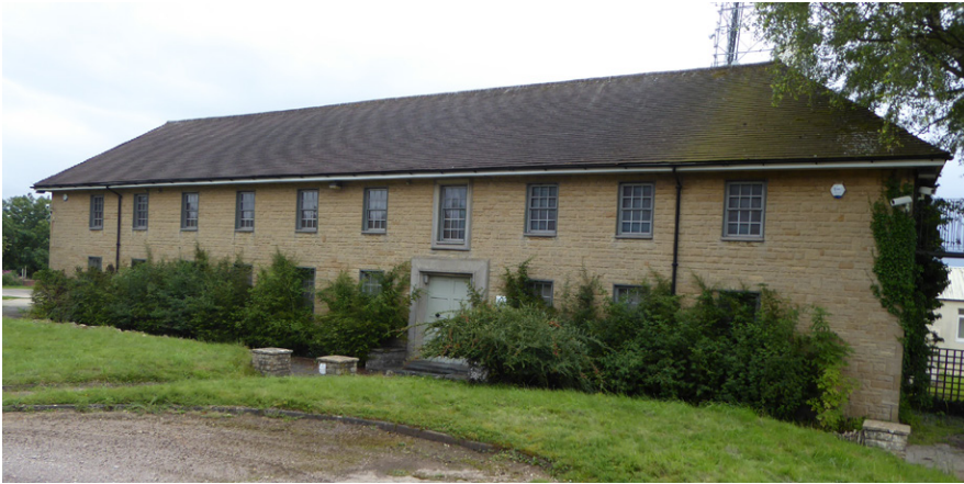
Figure 29. Birdlip radio station, showing the air traffic control room (a) built c. 1960, an aerial view taken in the early 1960s from the Guild of Air Traffic Control Officers' Archive ( https://atchistory.wordpress.com ) and some of the surviving wartime buildings.
